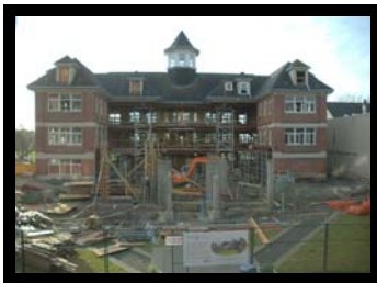
School House Construction
